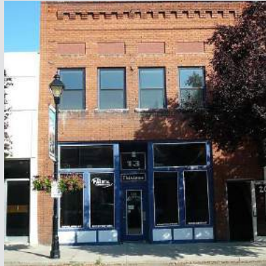
Building entrance flush with sidewalk - barrier-free
