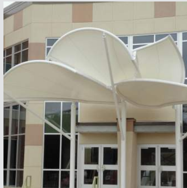
Highly intricate awnings typically do not match historic brick buildings. Awnings should subtly complement the building fabric not detract from it.
