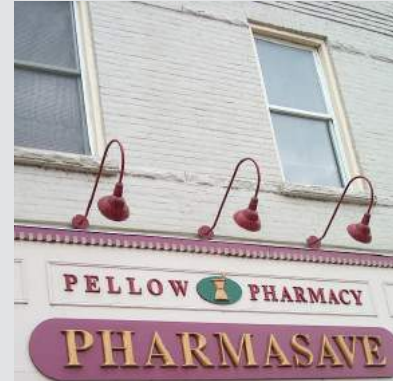
Traditional 'Gooseneck' lighting painted to match building colour scheme.
