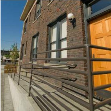
Concrete ramp with guardrail provides access to historic building. Note colour of handrail.
