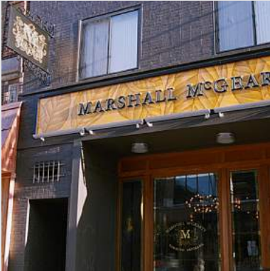
Small spotlights highlight sign and entryway. Note decorative sign board and block metal letters.
