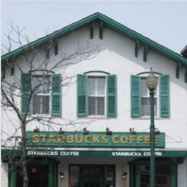
Wood shutters proportionate to the windows maintain the historical character of the building.
