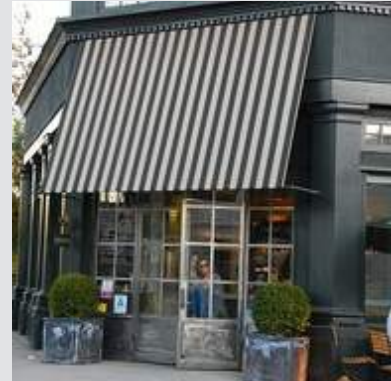
As an acceptable awning alternative, steep pitch awnings respect sight-lines on street corners and may screen unsightly building faces.
