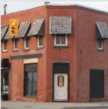
Use appropriate quality materials and ensure the use of materials that wear and weather well and reflect well on the building.
