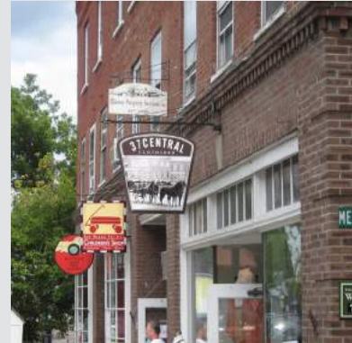
Custom decorative metal arm with hanging sign easily read by pedestrians. Note continuity down street.
