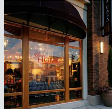
Natural wood detailing around windows and doors creates an inviting street presence.
