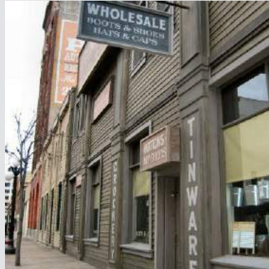
Wood siding can be used both horizontally or vertically, but consistency is key.
