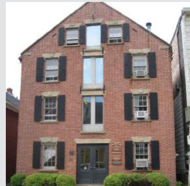
Unappealing and inappropriate shutter style.
