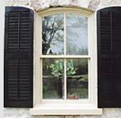
Contrasting black wood 'louver' style shutters with curved top provide a good fit for the window.
