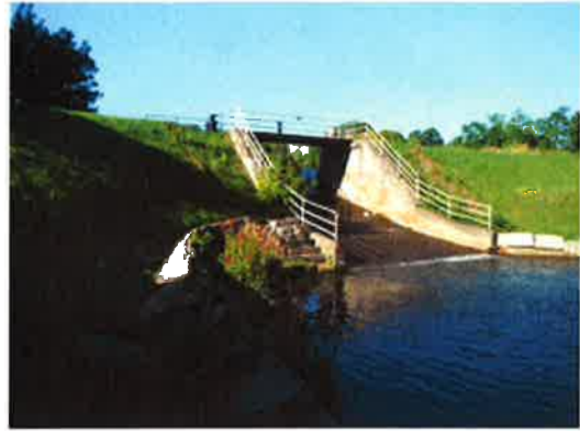
Spillway (Looking Southwest)
