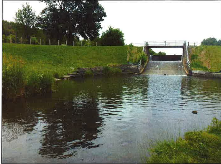
View of dam/spillway
