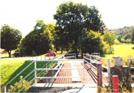
Steel Pedestrian Bridge (Looking East)
