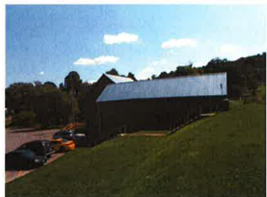
Stabilizing Berm (Looking East)
