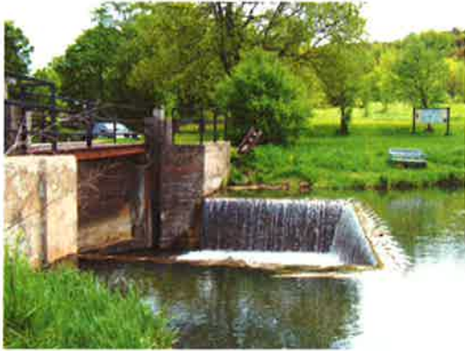
U-Shaped (Overflow) Weir (Looking East)
