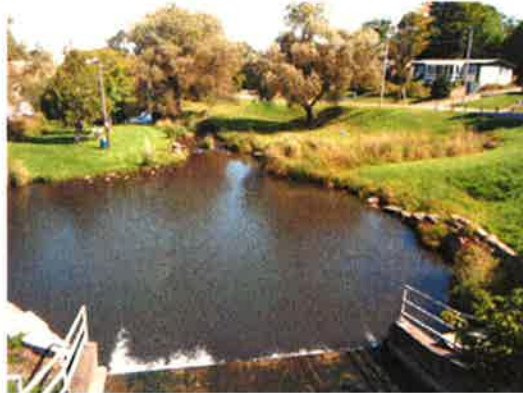
Plunge Pool and Island Below Spillway (Looking North)
