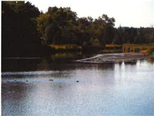
Sediment Accumulation (Upper Headpond) (Looking South)
