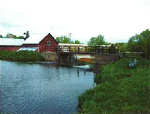
Upstream Dam Face (Looking Northwest)
