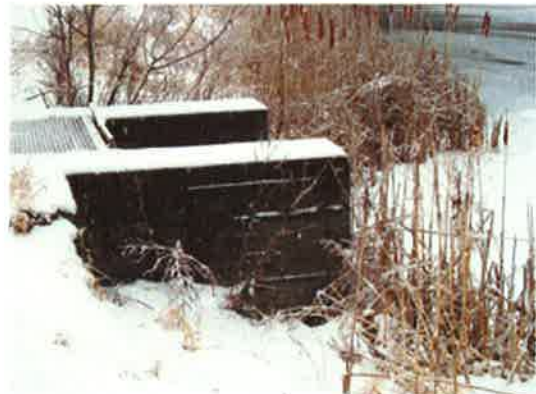
Penstock Intake (To Needler's Mill) (Looking East)
